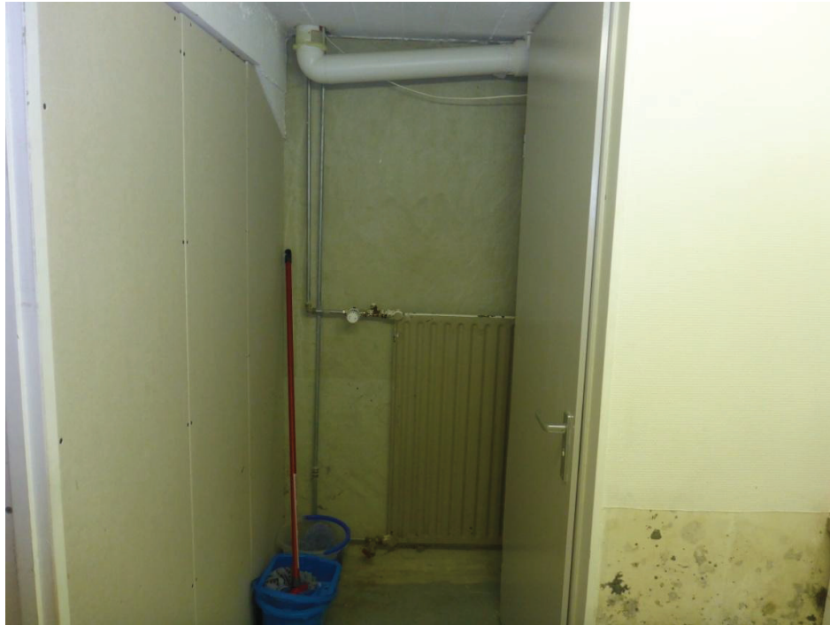
Detailfoto 3: toilet in de kelder
